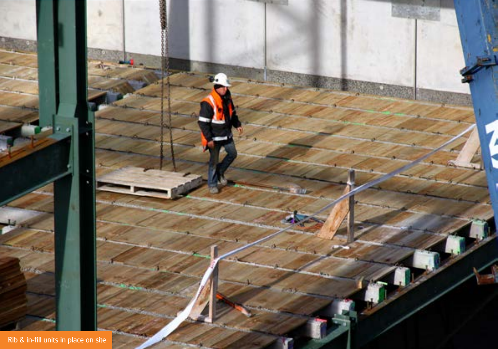
Rib & in-fill units on a Stahlton yard
