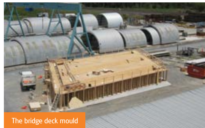
The first bridge deck unit being cast
