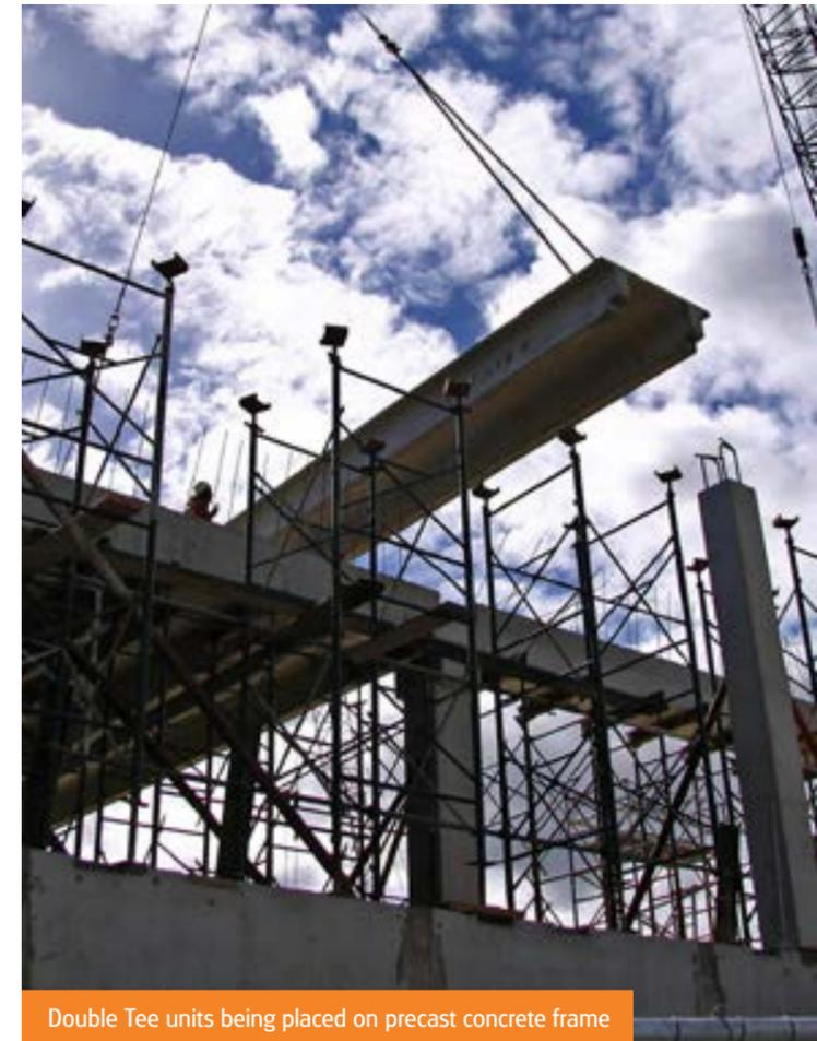
Double Tee units being placed on precast concrete frame
