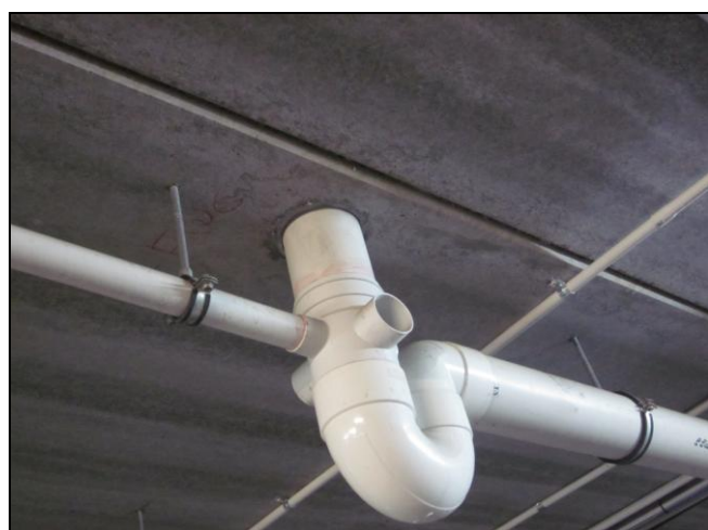
Figure 1: Plumbing penetrations in Hollowcore
