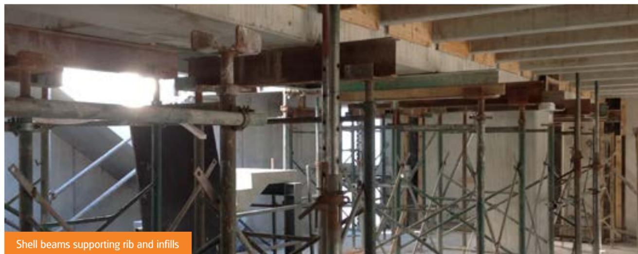
Shell beams supporting rib and infills
